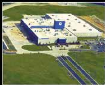
PAGELAND, SC Bronze Foundry and Manufacturing Plant
